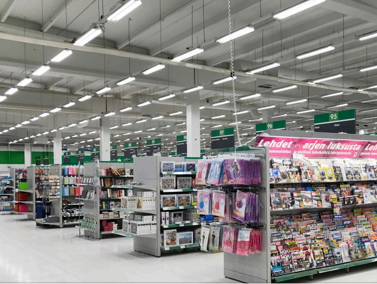
Total of 2490 fluorescent tubes were replaced with Valtavalo 28W G4 LED tubes in the Prisma department store in Kajaani, Finland during February-March 2017. This means an energy saving of approx. 60% as well as increase of the amount of light by dozens of percents. The new lighting is also flicker free. **A**PRISMA
