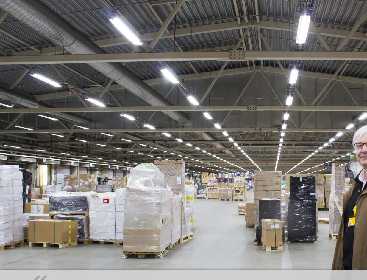
The lighting of the Vantaa terminal was updated with Valtavalo's LED tubes as couraged by good experiences gained from the lighting update of Turku warehouse. Various measurements were executed in the premises by a technical maintenance professional before and after the installation. In addition to the significant 60% energy savings, we noticed that the LED tubes achieve 25% higher illuminance than the T8 fluorescent tubes that were previously used in the premises.
